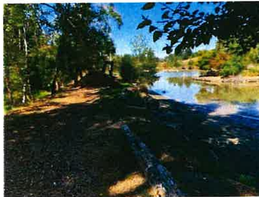
Looking at Drained Water surface; Excavated pit on 'Retaining Dike'
