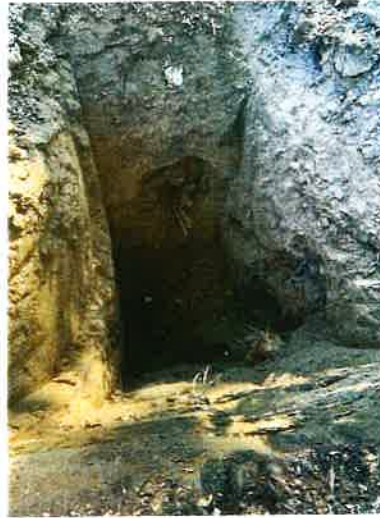
Top View of Exploratory Pit on 'Retaining Dike'
