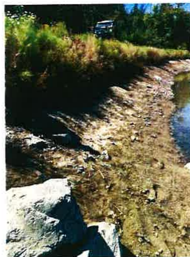
Southwest 'Retaining Dike' at Location of Proposed Rip Rap
